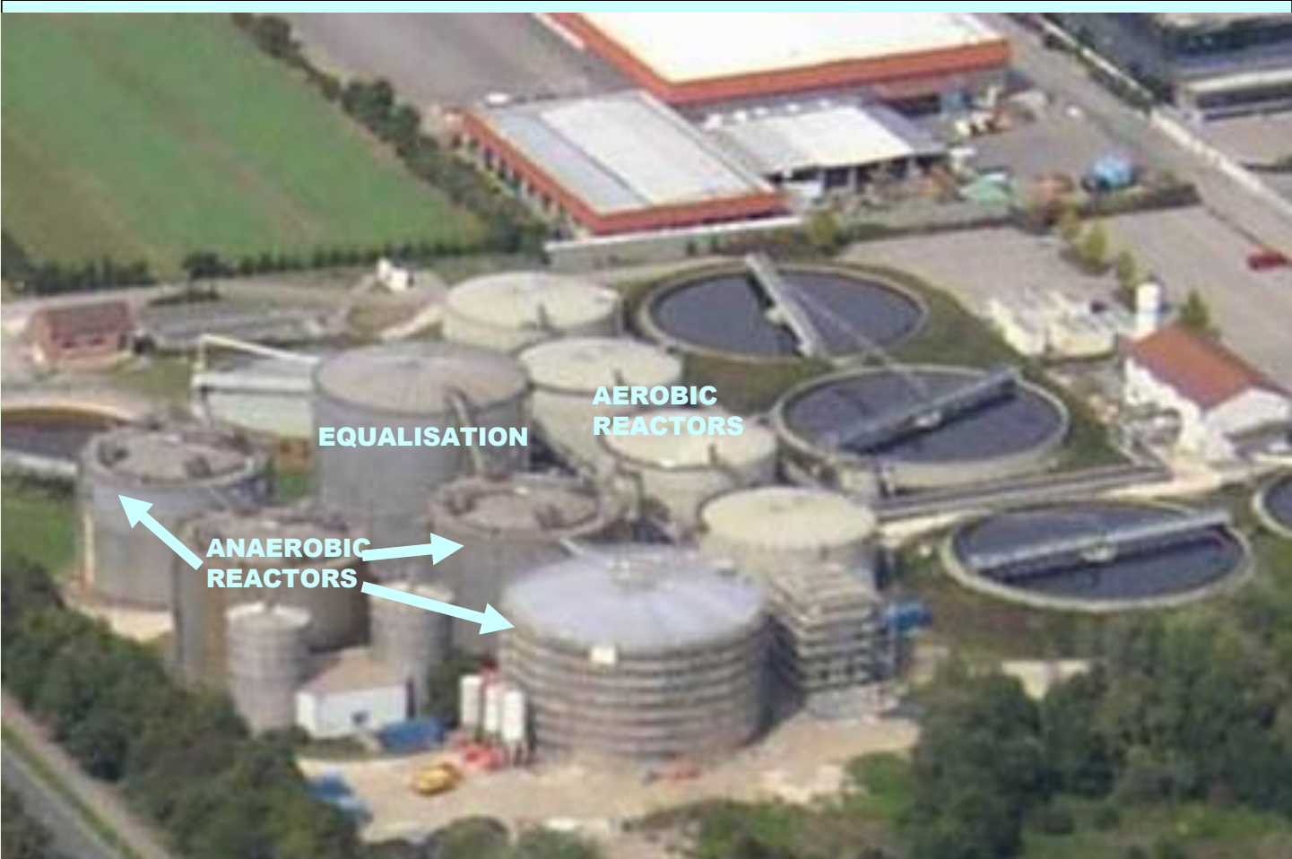
Anaerobic-aerobic WWTP for the treatment of toxic pulp mill effluents by microorganisms fixed on LEVAPOR-biocarriers
